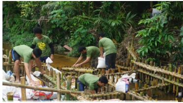
Making dam with natural materials
