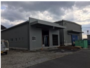
Cutting facility in Kamiura
