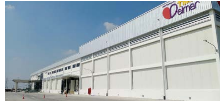
Completion of construction in May 2020
