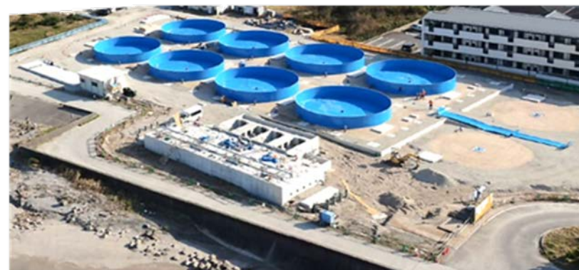
Verification test facility (Yonago, Tottori)
