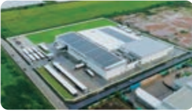
Solar power generation facilities (Thai Delmar Co., Ltd.)
