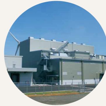
Fine Chemicals General Factory Kashima Pharmaceutical Factory
