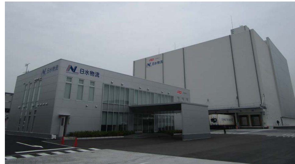
Nissui Oosaka-Maishima Logistics Center (Plant capacity : Approx. 25,400 ton) Completion of construction in March 2016 and start running in April 2016
