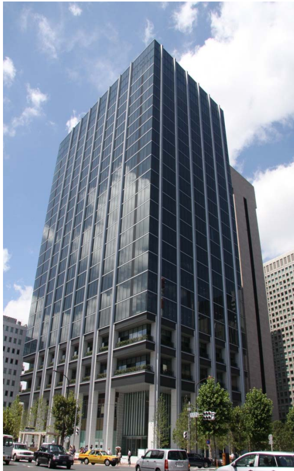
Exterior appearance of the building
