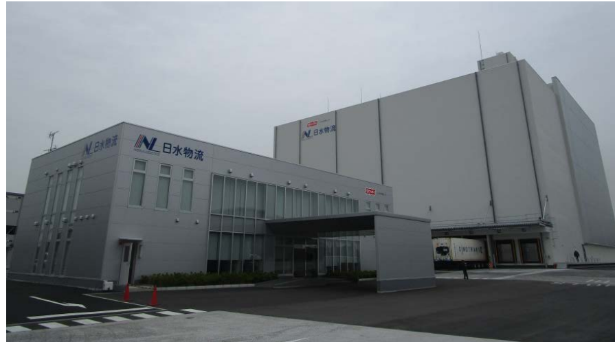
Nissui Osaka-Maishima Logistics Center (Plant capacity : Approx. 25,400 ton) Completion of construction in March 2016 and start running in April 2016
