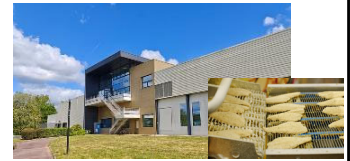
Europe: Expanded Plant (Commercial operation from 1H FY2026)
