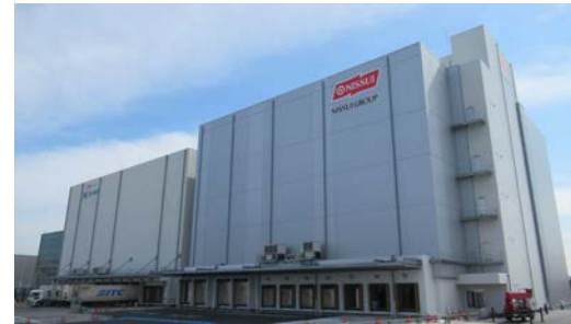
“Osaka Maishima Logistics Center No.2”, Nissui Logistics Completion of construction on March 26, 2020 Start operation on April 1, 2020, Capacity : 24,887 M/T
