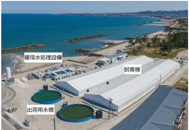
Land-based farming facilities for chub mackerel Complete construction in May 2020
