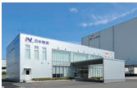
Osaka Maishima Logistics Center, Nissui Logistics Corporation
