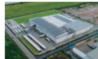
Solar power generation facilities (Thai Delmar Co., Ltd.)
