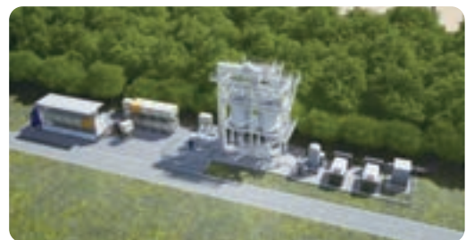
Land-based silos used in a remote feeding system Source: Nippon Steel Engineering Co., Ltd.
